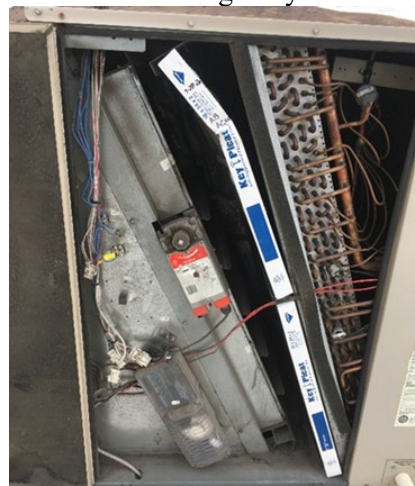
Figure 4. Picture of a filter that is not seated correctly.
